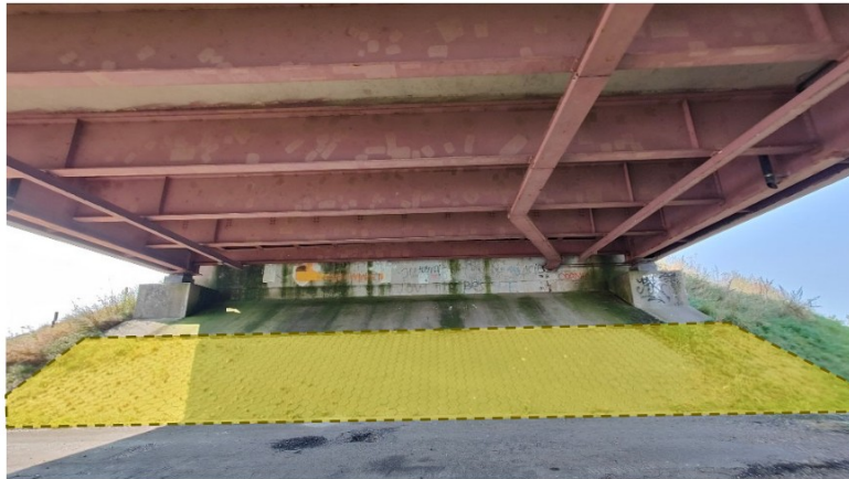
STP 04 (LH WEST)
