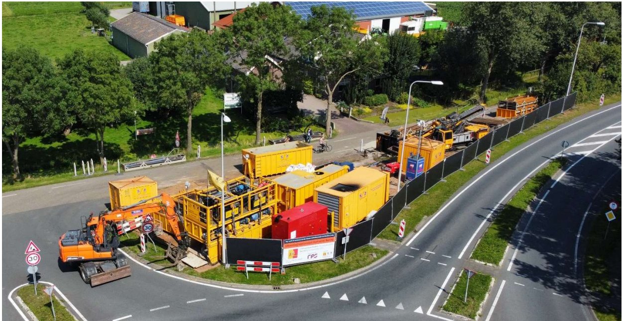
80-ton drilling rig
