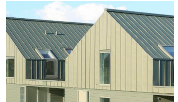
houtstructuren dmv felsbanen
