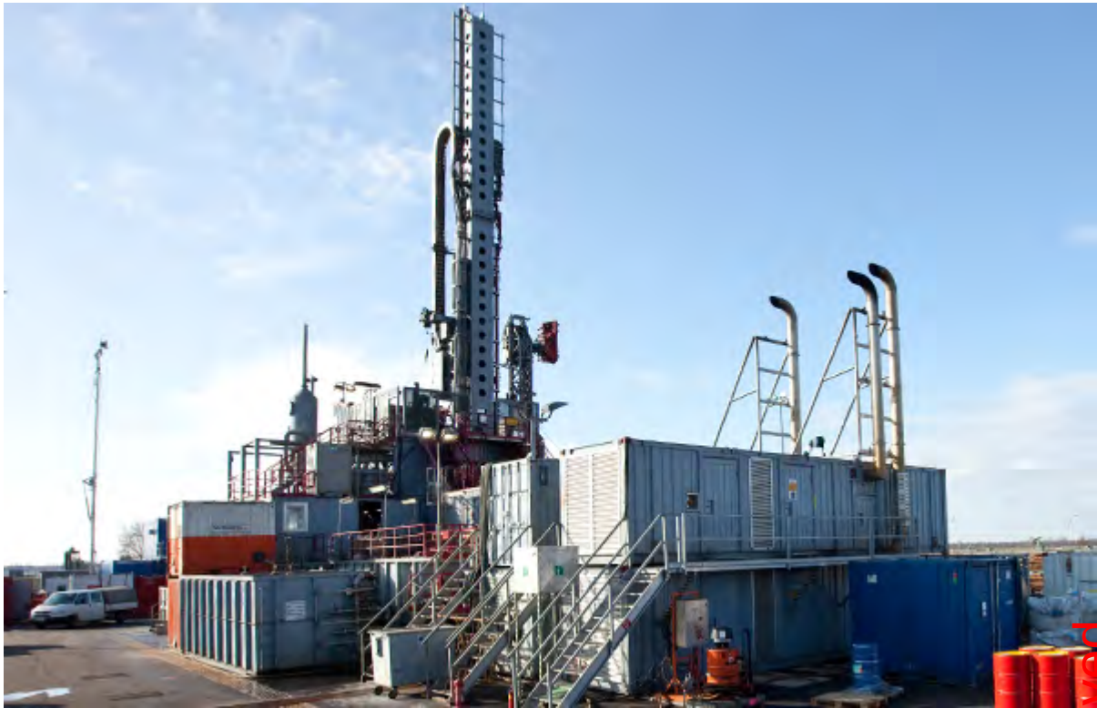
Figure 5.3: Photo of DrillTec VDD 370 rig
