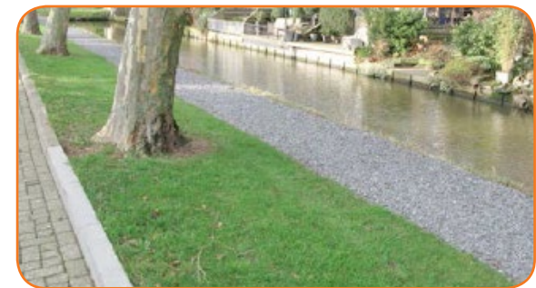
Boomvak in berm
