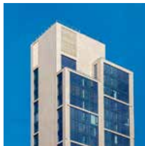
Luchtzuiverende materialen Skidmore, Owings & Merrill, 570 Broome New York
