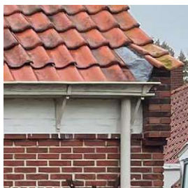
HOUTEN PLANK + ZINKEN GOOT
