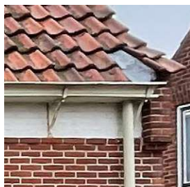
HOUTEN PLANK + ZINKEN GOOT
