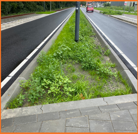
Water infiltratieberm (Bronvermelding: RHDHV)
