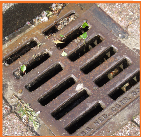
Putdeksel (Bronvermelding: GAW | stichting RIONED)
