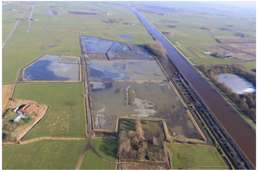
Baggerdepot Garmerwolde (foto: Noorderzijlvest)
