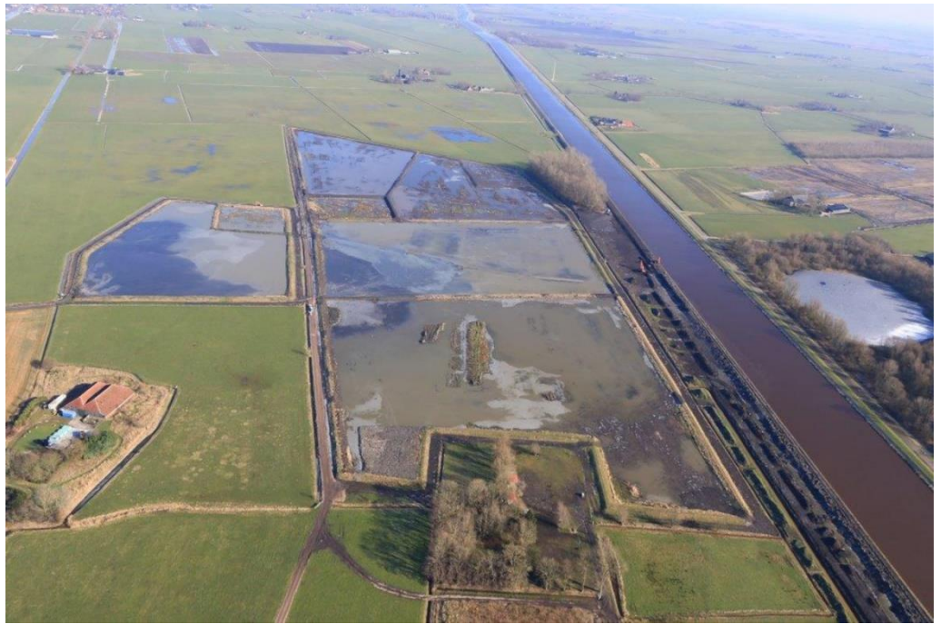
Baggerdepot Garmerwolde (foto: Noorderzijlvest)
