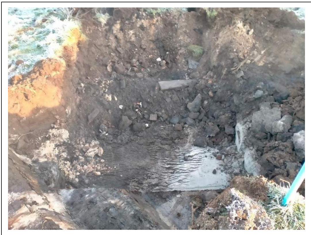
Foto 2. Ontgraving PAK-spot
