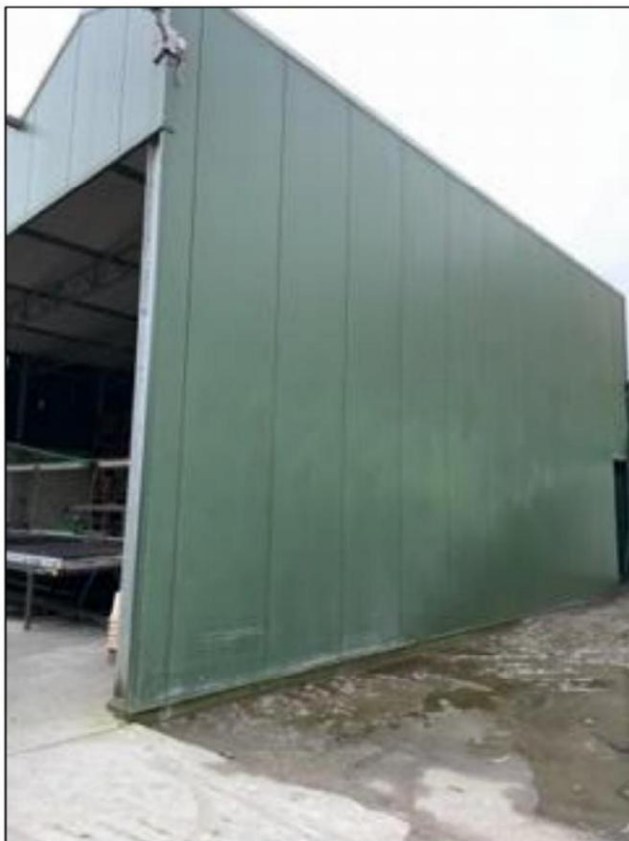
Afb 16: Sandwichpanelen dicht
