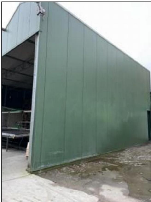
Afb 16: Sandwichpanelen dicht
