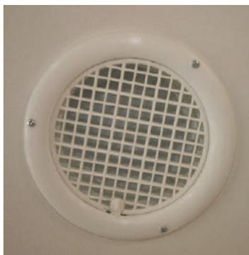
It is important that all ventilators are kept unobstructed, especially at floor level. Remember that gas is heavier than air; therefore it is essential that the ventilation provided is kept clear to ensure that no risk to life occurs due to faulty gas appliances. All ventilators should be cleaned and checked to ensure they are unblocked. All blocked ventilators should be cleared to ensure they allow a free passage of air.
