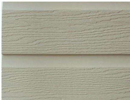
It is recommended that Canoxel cladding be periodically cleaned. This normally would be carried out using a soft brush or sponge along with a mild detergent mixed with water. This cleaning is, in fact, a condition of our warranty and the consequences from dirt and mildew
