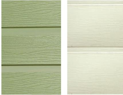
In most cases normal rainfall is sufficient to keep it clean, but if your vinyl cladding should need cleaning, an occasional wash with clean water using a garden hose (not a jet wash), with a soft bristled brush is ideal for this purpose.
