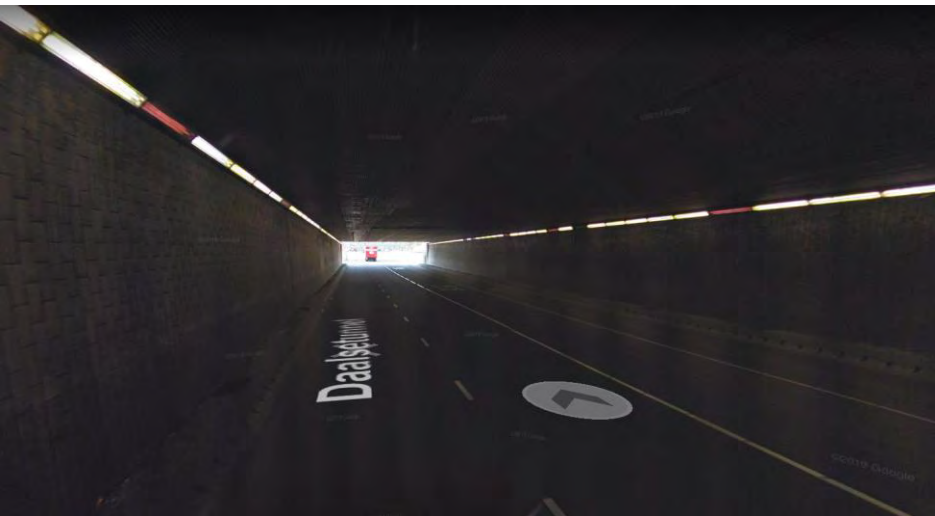
Situatie in tunnel
