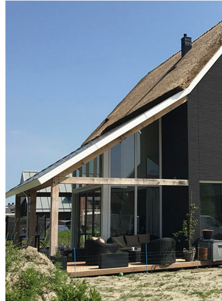
Gebroken dak
