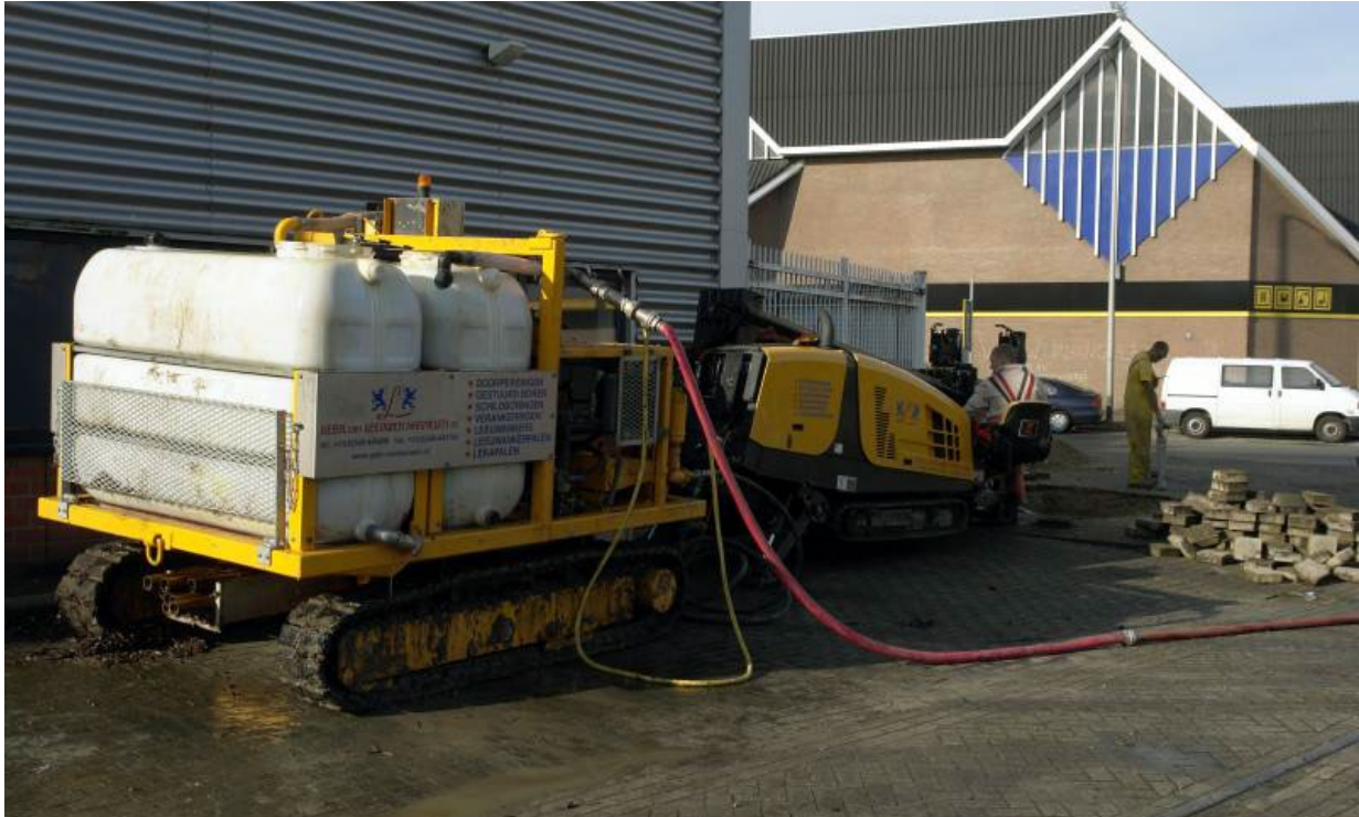
DitchWitch rig and mobile mix &amp; pump unit at industrial estate in Utrecht (NL)
