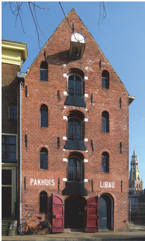
Pakhuis Libau in Groningen
