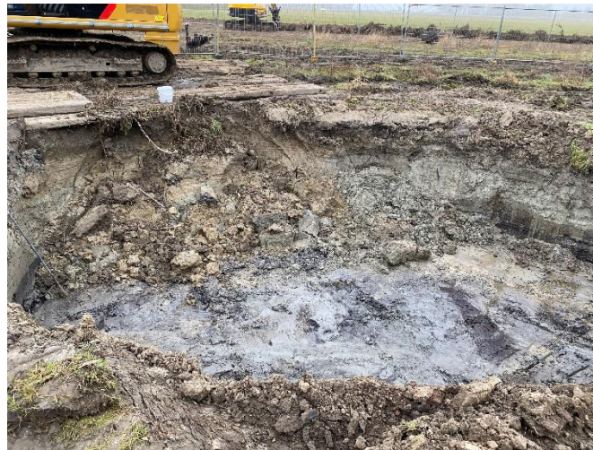
Foto 29: Ontgraving oliespot (5)
