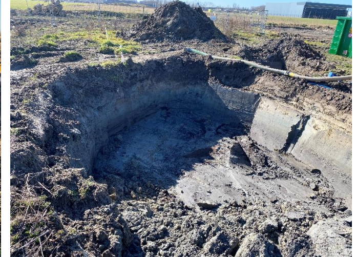
Foto 27: Ontgraving oliespot (3)
