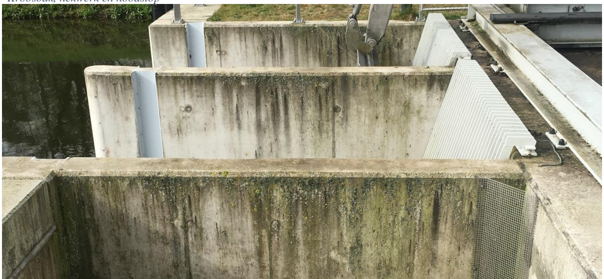
Schotbalken, middenwand, krooshek
