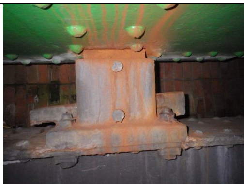
Detailfoto 9: Oplegging1 links
