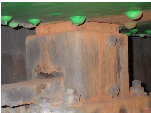
Detailfoto 12: Oplegging 2 links
