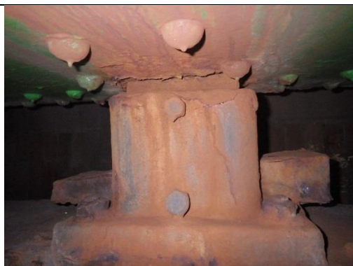
Detailfoto 13: Oplegging 3 links
