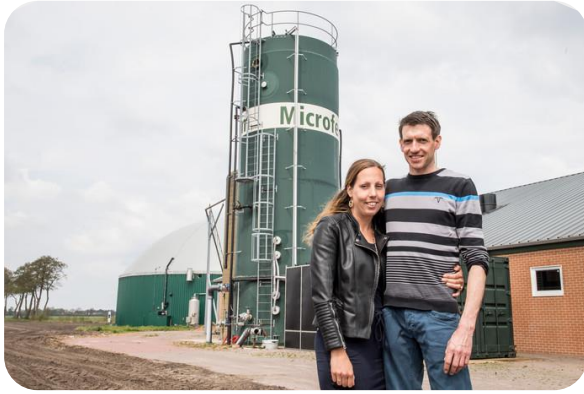
Fig. 5 Biovergister in Langeveen 6
