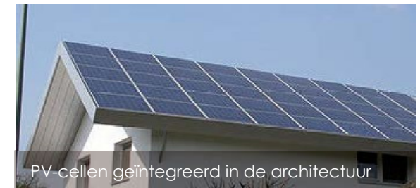
PV-cellen in nette, regelmatige vlakken
