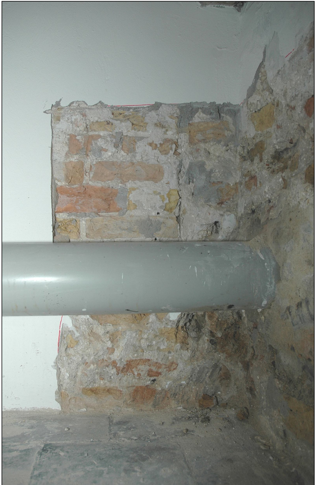
[ [9] De rechter dagkant was in de kelder terug te vinden, linksachter, 2009
