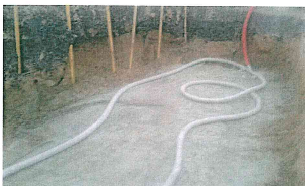
Foto drainagestreng in ontgraving
