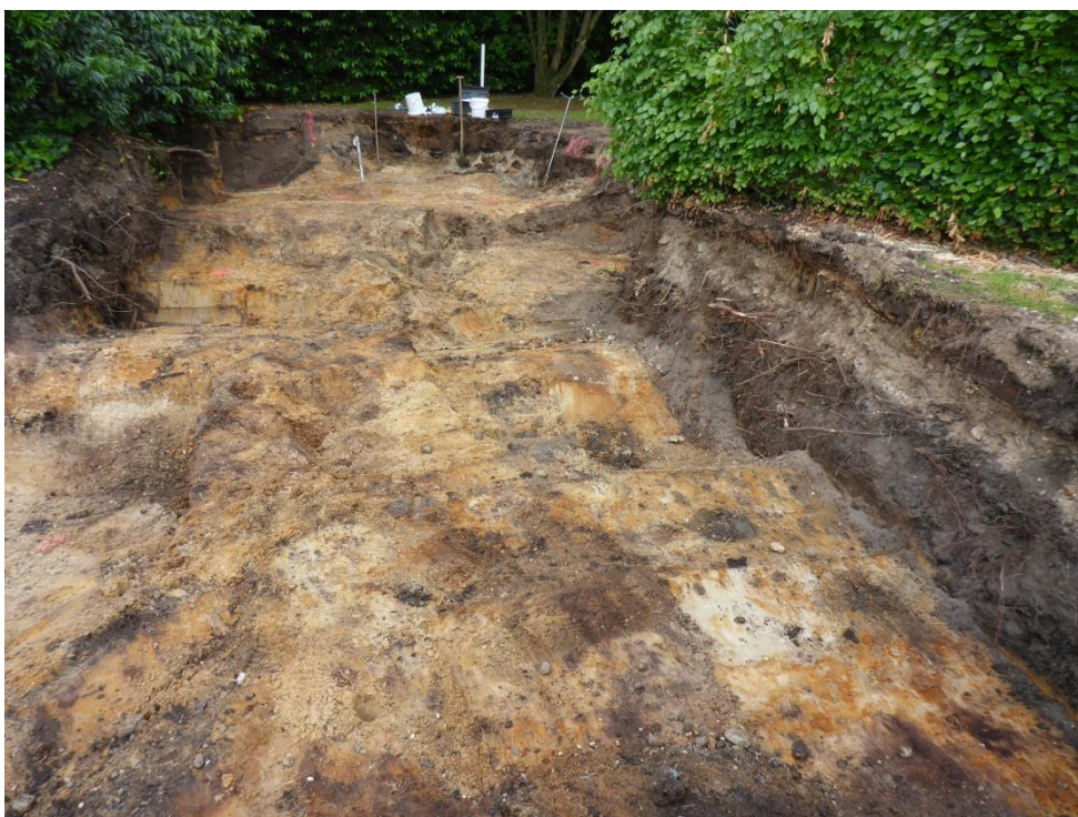
foto 24: P1050910.JPG: Tussenstand ontgraving.
