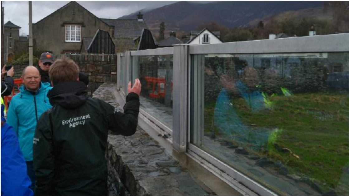
Figuur 7: Impressie glazen waterkering
