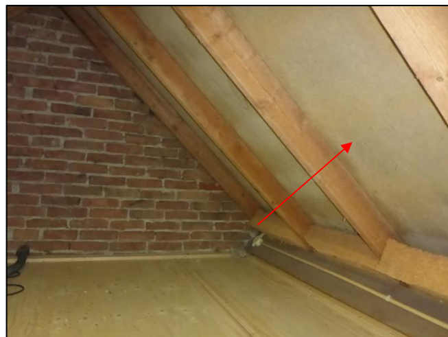
Foto 8: Woning: Dakbeschoot (M01AA)
