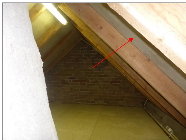
Foto 6: Woning: Dakbeschot (M01AA)
