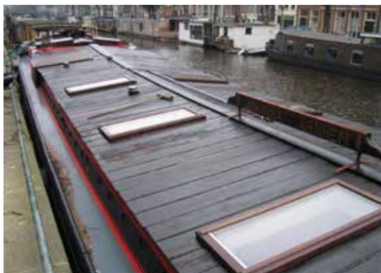
Dakramen in houten luikendak
