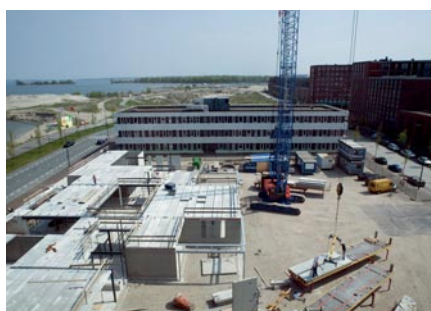
Brede School Archipel-Poseidon in aanbouw
