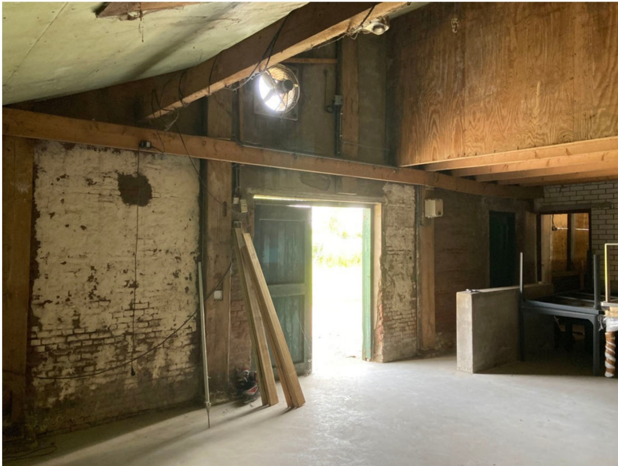
Turfloods (linker travee), verdieping secundair ingebracht
