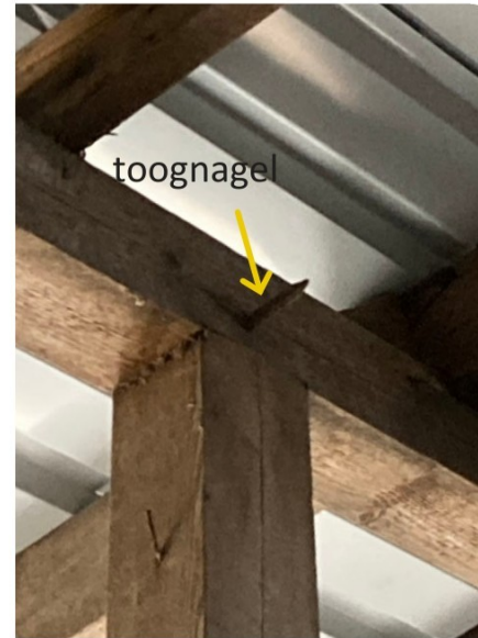
Detail toognagel van pen-en-gatverbinding
