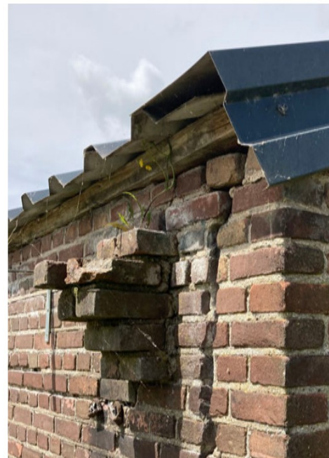
Gemetselde console dakgoot
