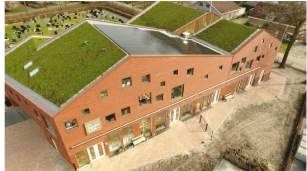
Figuur 2-2 Groendak MFC Rottevalle [ https://www.climatescan.org/projects/16844/detail ]
