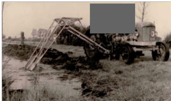
De Ridder slootreinigingsmachine met aandrijving door middel van lieren. Hydrauliek was nog geen gemeengoed in die tijd. Deze foto is van omstreeks 1960. The Ridder ditch cleaning machine driven by means of winches. Hydraulics were then not common yet. This photograph is approximately from 1960.
