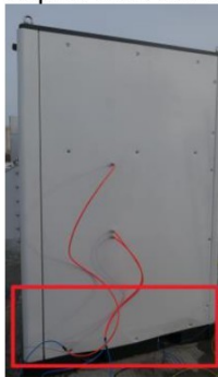
Figure24 Deformation of right plate
