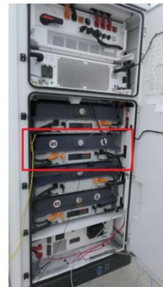
Figure10 The pack installation in test
