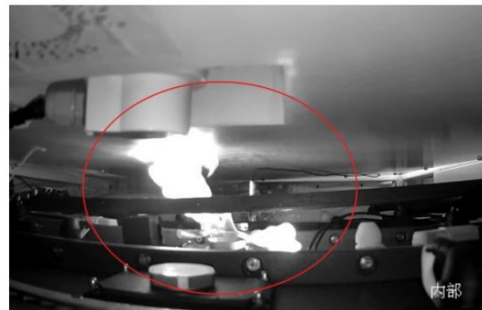
Figure41 Visible flame appears after explosion
