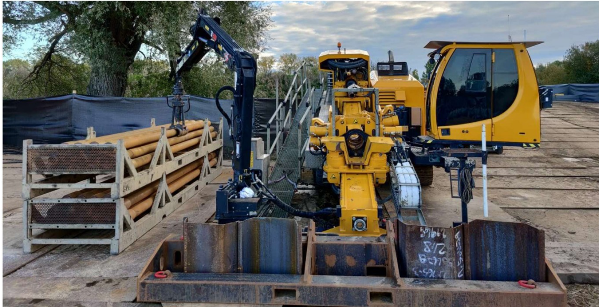
50-ton drilling rig (10-2020)
