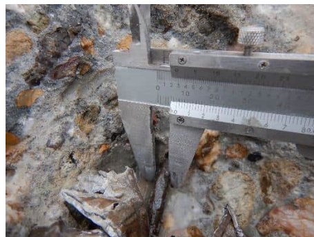
Foto 6.64: Diameter 3 e laag (Ø7 mm).
