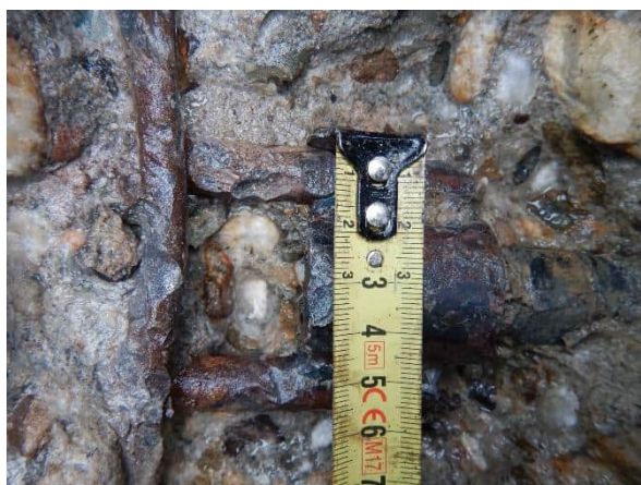
Foto 4.14: Diameter lasbus (± Ø3 cm).
