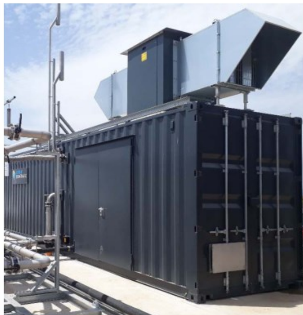
Biogascompressor in membraancontainer
