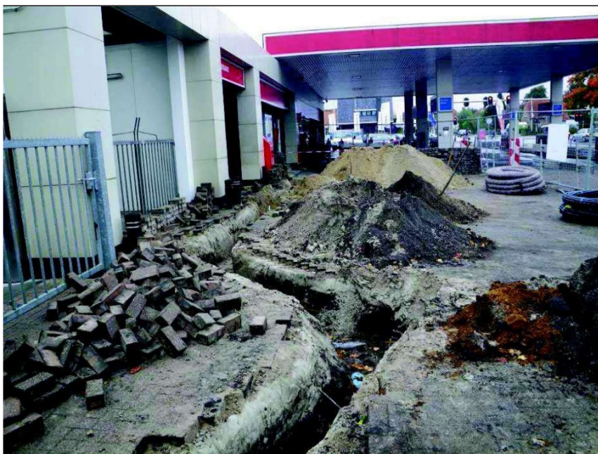
Figuur B3.8 Aanleg leidingen en BLE drain nabij tankstation
