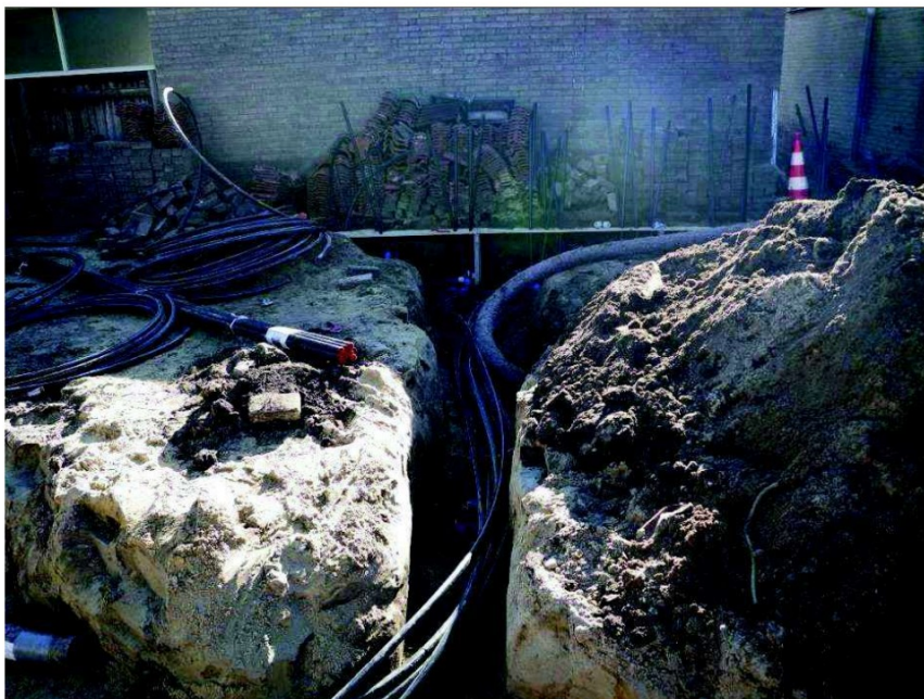
Figuur B3.6 Leidingen en BLE drains nabij aanstuurunit
