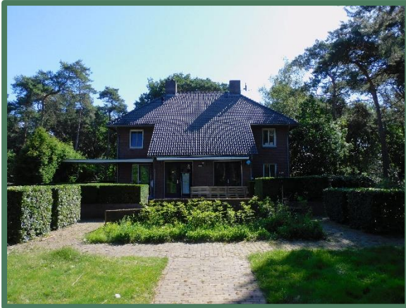
Te slopen woning
