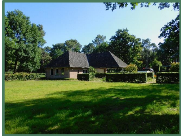
Te slopen garage
