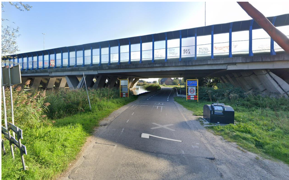
Figuur 1.5 Viaduct A9 over de Bullewijk (Bron: Google Maps)
