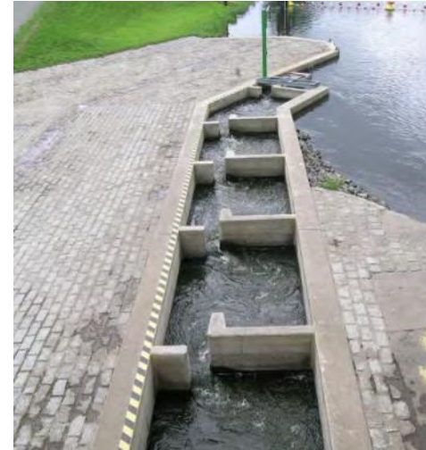
Vertical slot vispassage LUGV Brandenburg, Potsdam (2007)
