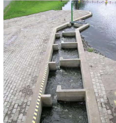
Schlitzpass (Vertical Slot) LUGV Brandenburg, Potsdam (2007)
