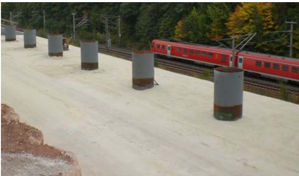
Photo 1: Steel casing installed into the geogrid reinforced earth structure
