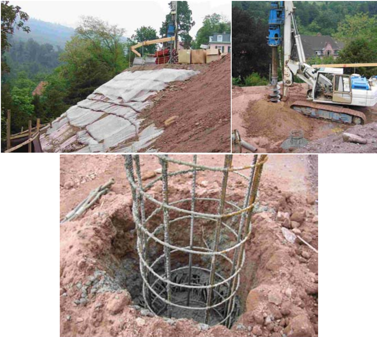
Photo 3-5: Geogrid reinforced slope, drilling machine and reinforcement for the concrete column
