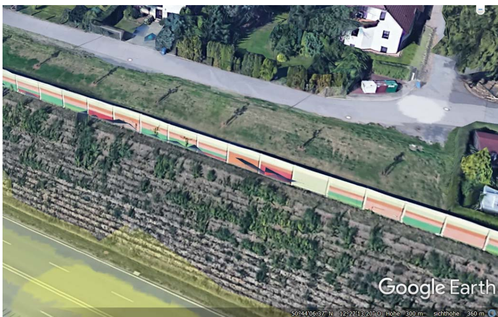
Photo 2: Reinforced slope with noise protection wall on top, Google Earth screen shot
